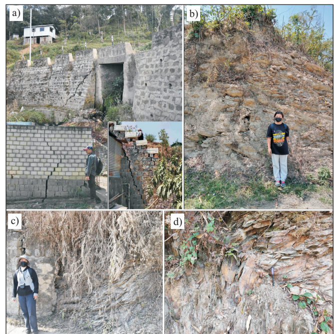
Fig.2. a) Tension fractures observed in structures indicating movement in the area, b) Crumbled weathered shale exposure in the area, c) Partially weathered shale in the study area, d) Disang shale intercalated with siltstone.
